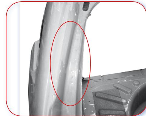
17.2.D Good example. The drain channel is made out of one piece, joining the outer and inner panel.
